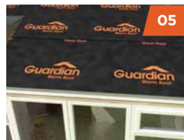
05 Breathable waterproof membrane is laid over the ply-wood and secured in place.
