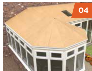
04 Exterior grade ply-board is fixed to the rafters.
