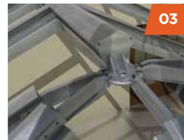
03 The aluminium rafters, ridges and wall plates are fitted and the spider arms are secured to the spider bracket.
